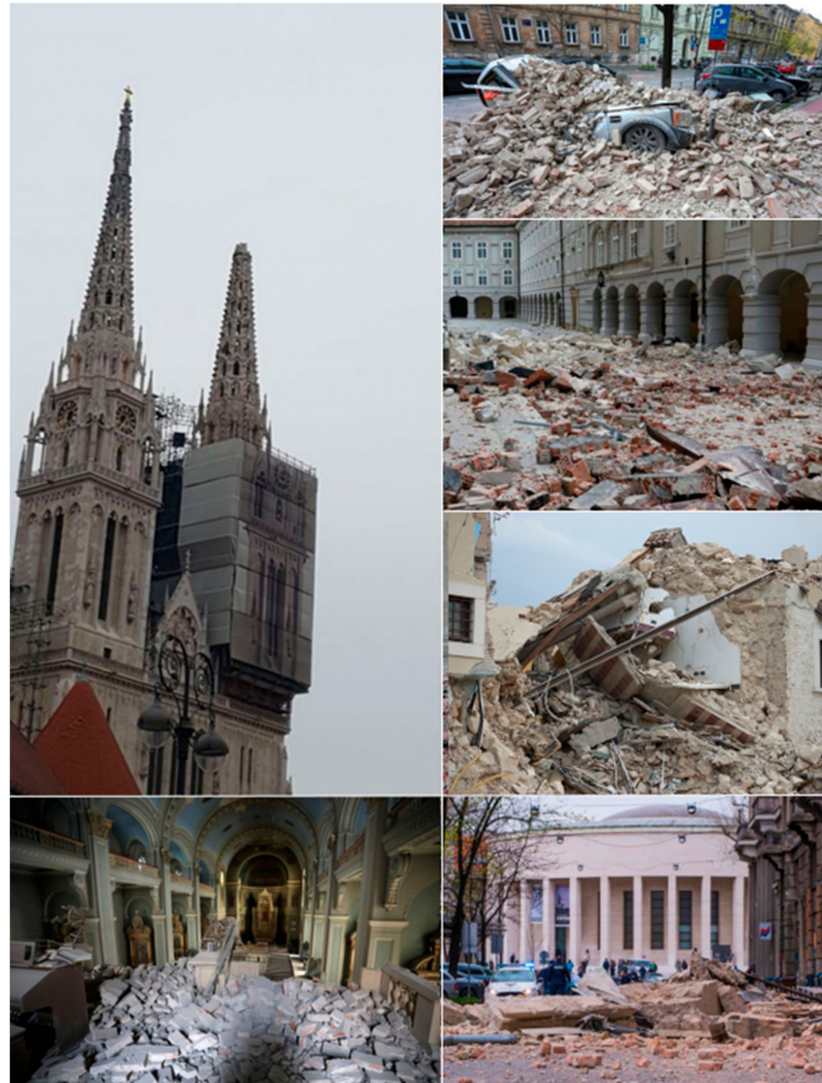
Figure 6. Photos of damage in Zagreb caused by the 22 March 2020 earthquake.
