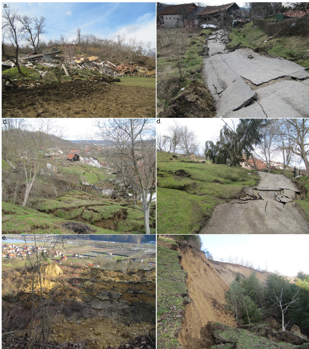
Figure 3. Hrvatska Kostajnica landslide damages: (a) completely destroyed houses; (b) completely destroyed road and damaged objects; (c) cracks and heavy terrain deformations; (d) flow like deformations on terrain surface; (e) view from main scarp toward flooding Una River; (f) landslide main scarp—almost 30 m at the highest point (photos by Croatian Geological Survey (CGS), day after the event, 14 March 2018).
